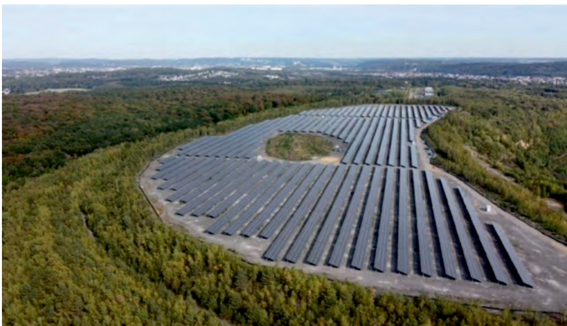
Fig. 4. Lorraine Basin — France – installation of PV on existing coal dump- Wendel (Source: Luxel)
